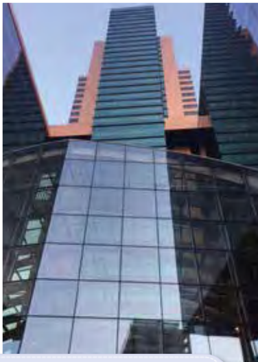
Santiago Marriott Hotel solidly built to withstand seismic activity
